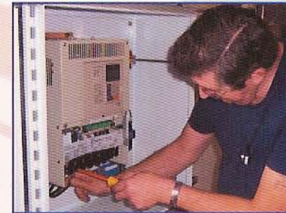
In-House Electrical Line Integration
